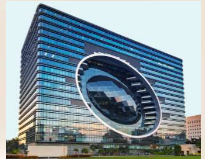
25 South – Residential The Capital - Commercial
